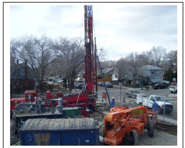
Photo: Setting Casing for the Well
