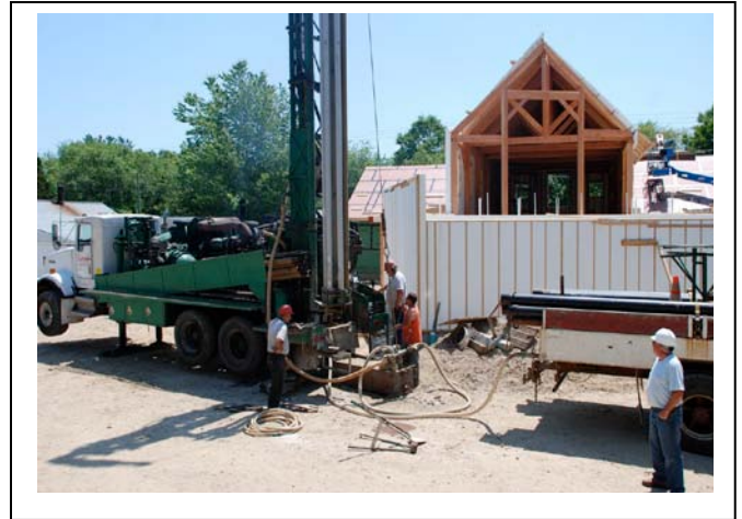
Photo: Installing Geowell at Wine Shop in RI
